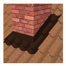
Fig 9.5.4 Gluing the roofing tape
