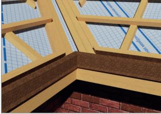
Fig 8.6.3 Eaves flashings
